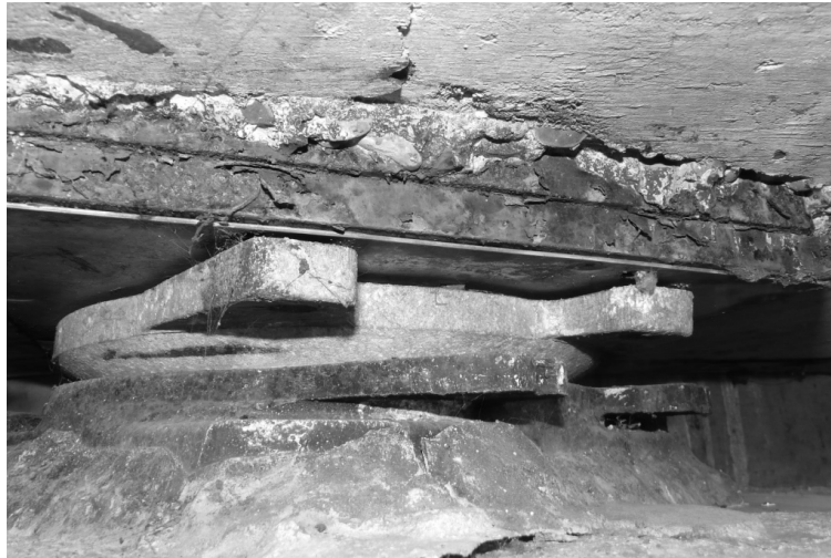
Vicarage bridge bearing
